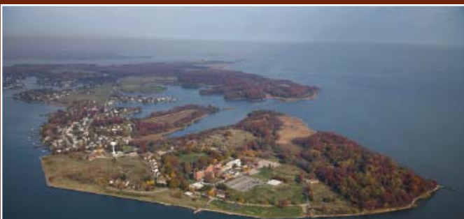
An aerial photo of the Bayside at Fort Howard project site.
