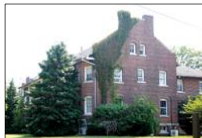
Old Fort Howard VA Medical Center buildings like this one will be preserved and used anew at Bayside at Fort Howard. Photo by Marge Neal
